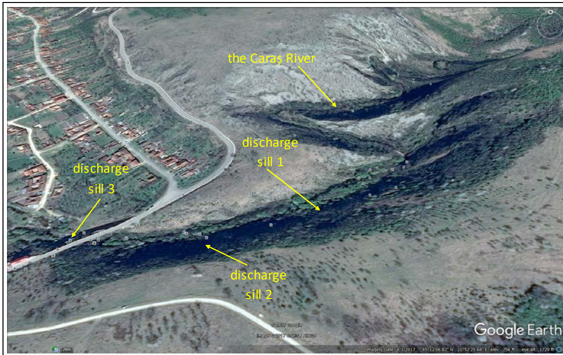
Figure 2: Position of Caraș River upstream of Carașova Village.
